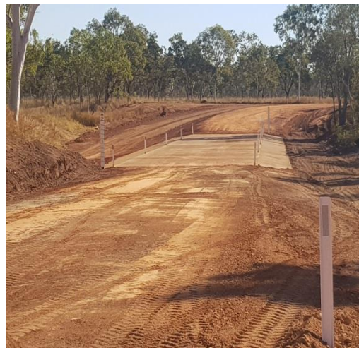
Construction of causeway at Hobbestrup Creek, Robinson River Road
